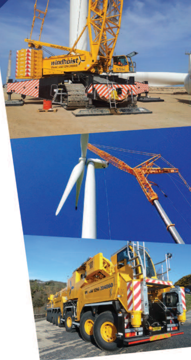
Top photo: Demag CC2800NT, erecting Siemens turbines, Tarfaya, Morocco
