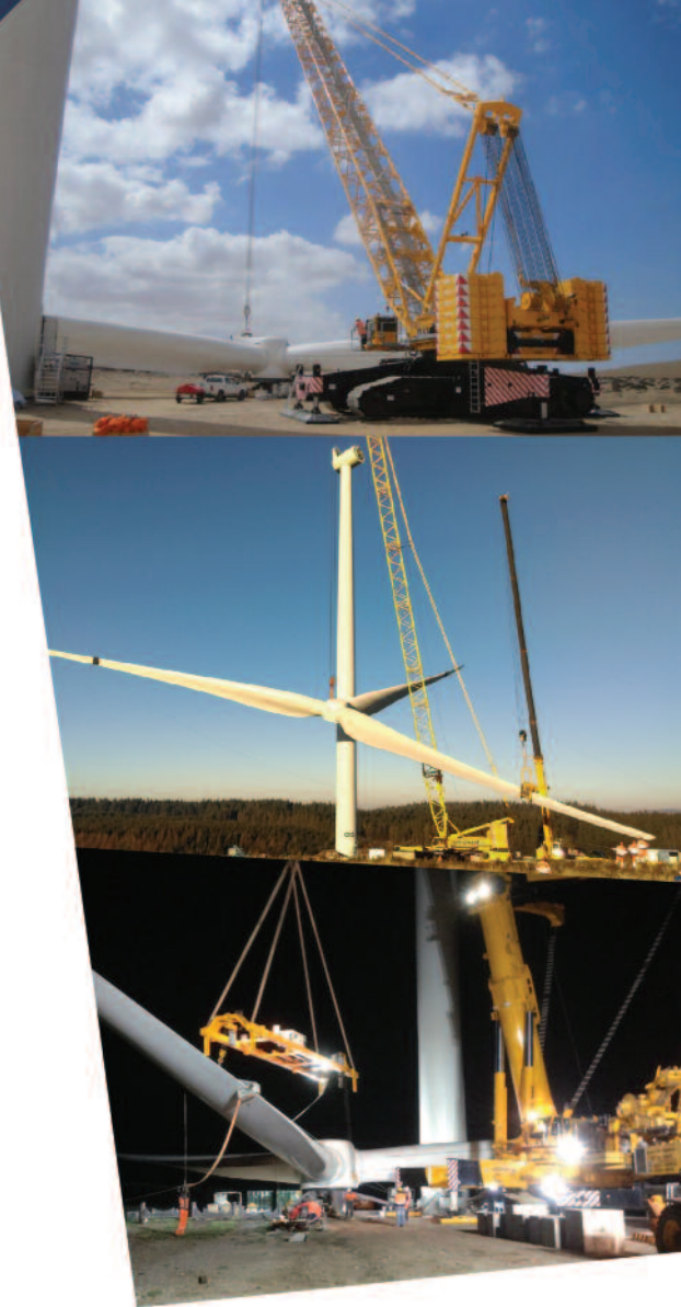
Middle photo: TC2800 & LTM1130 erecting Siemens turbines, Pen Y Cymoedd, UK
